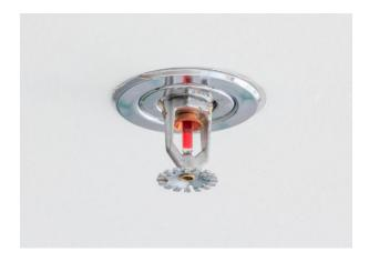
The proper functioning and activation of fire sprinklers is essential to ensure that the fire is quickly controlled and to prevent fire development and spread from affecting the safety and security of persons and facilities. In Spain, fire sprinkler systems are required to undertake mandatory, periodic verifications and inspections.
