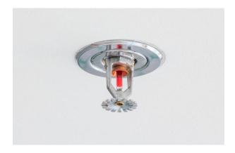
The proper functioning and activation of fire sprinklers is essential to ensure that the fire is quickly controlled and to prevent fire development and spread from affecting the safety and security of persons and facilities. In Spain, fire sprinkler systems are required to undertake mandatory, periodic verifications and inspections.
